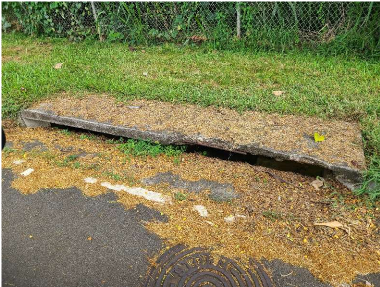
25. Typical Storm Drain Type 3
