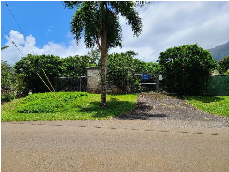
9. HHFDC Lot 59 booster pump station – TMK (1) 4-8-12:37
