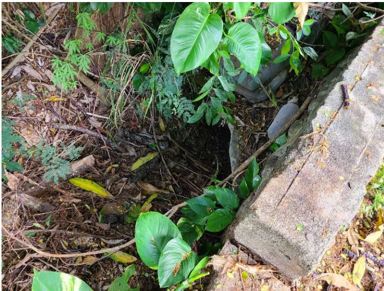
27. Typical Storm Drain Type 5 – riprap area behind drain
