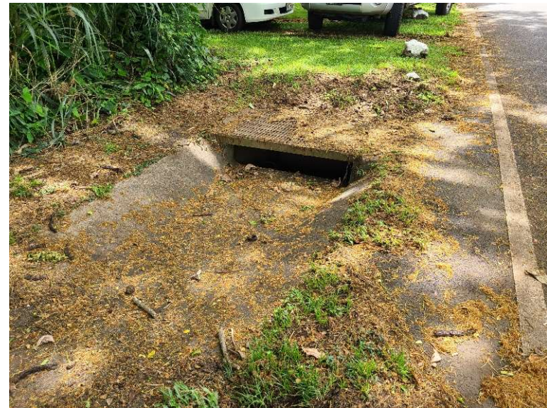
24. Typical Storm Drain Type 2
