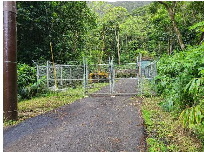
20. HHFDC State Well Site – Gate 4 Pump Site
