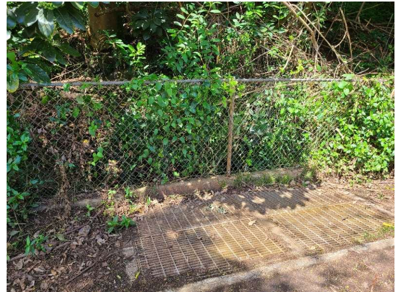
26. Typical Storm Drain Type 4
