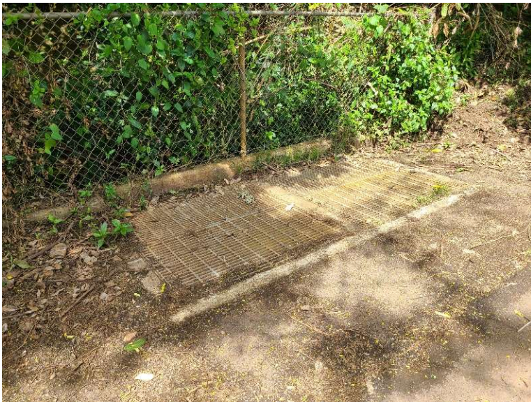
23. Typical Storm Drain Type 1
