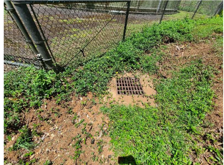
14. HHFDC Lot 77 water tank drain inlet – TMK (1) 4-8-12:44
