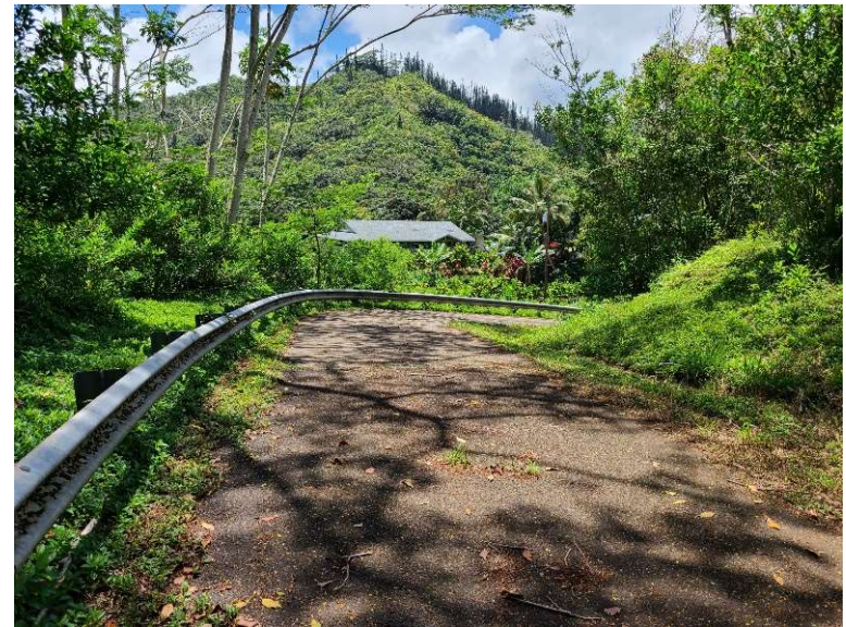
12. HHFDC Lot 77 water tank driveway – TMK (1) 4-8-12:44
